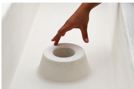
Water reserve system and overflow discharge
